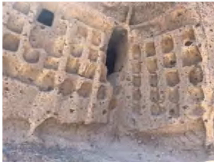
Figure 1. Differential erosion and missing part type deteriorations observed in the Şahmelik Tuff Rock Monument
