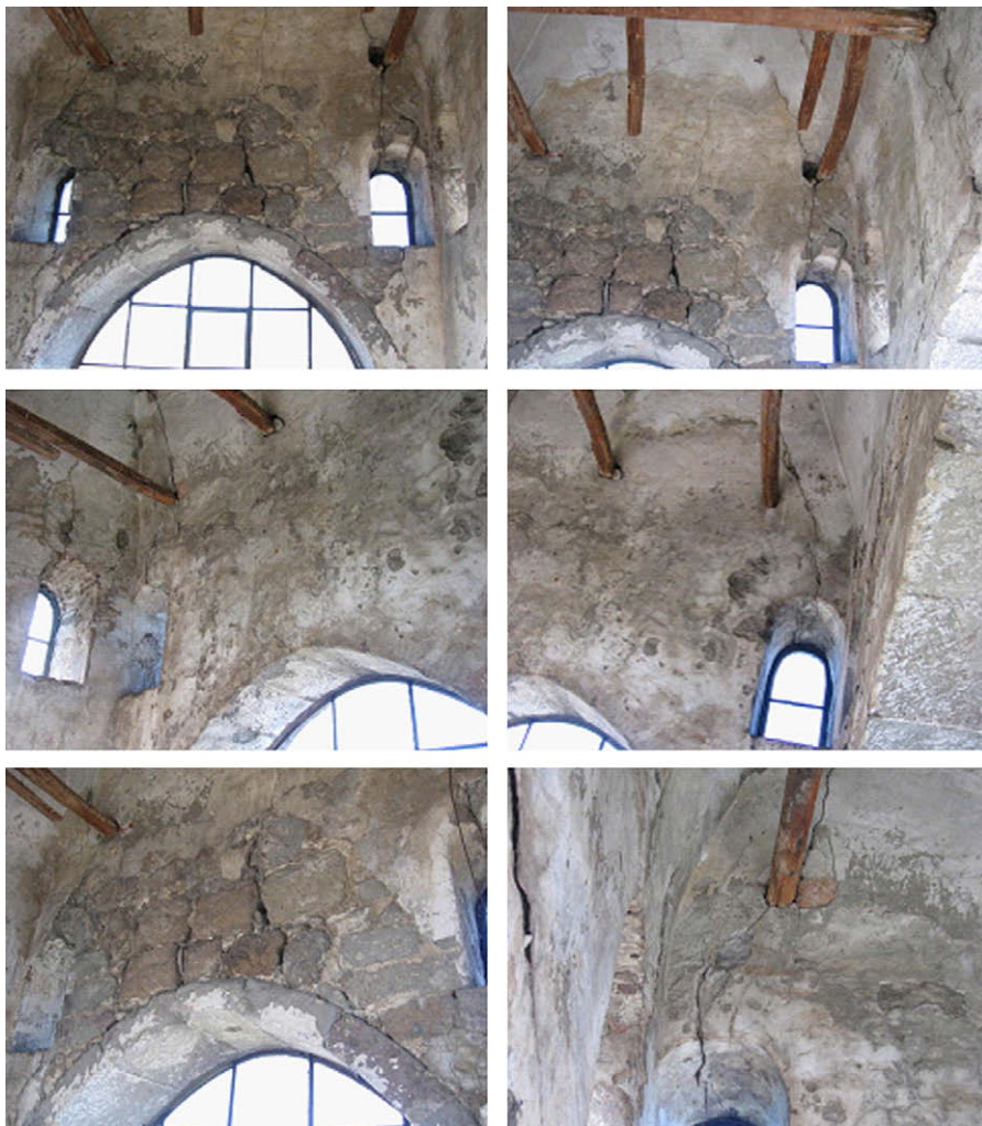
Fig. 10. Crack distribution in the bell tower, internal side of belfry (fourth storey).
