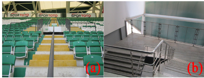
Figure 5. The Sample of Vomitories, Radial Gangways (a), and Stand Staircases (b) in Upper Stands.
